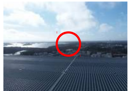
Photo from Battalion HQ roof top. Red circle highlighting the Company HQ location
