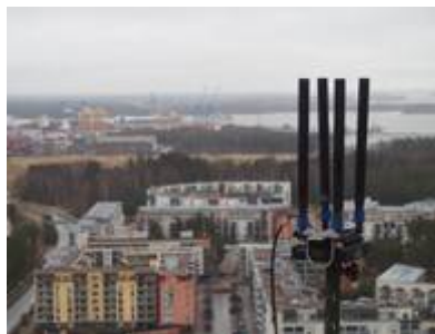
Silvus Streamcaster 4480 node at Cirrus building roof top.
