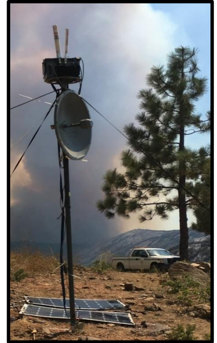
Solar powered mountain repeaters run indefinitely & reaches ~1.2 million acres
